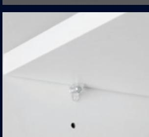
Shelves are made of 12 or 19 mm particleboard with melamine or high pressure laminate surface and all edges are sealed with 1 mm synthetic banding for optimal hygiene.
